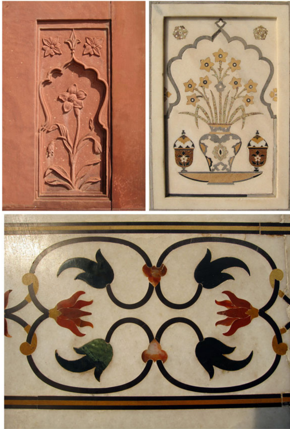
Fig. 10. Decorative changes (clockwise from top left). chini khana bas-relief in red sandstone; stone intarsia inlay in red sandstone; pietre dure inlay in white marble.
